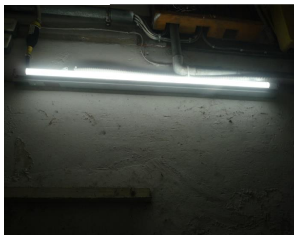
4' LED Tube installed in the staircase of the building
